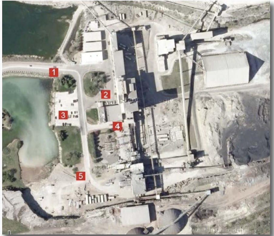
Figure 1. Photo of St. Marys Cement used in the containment control software. Each number correlates to a drain controlled by the system.
